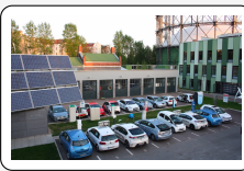
EV charging station
